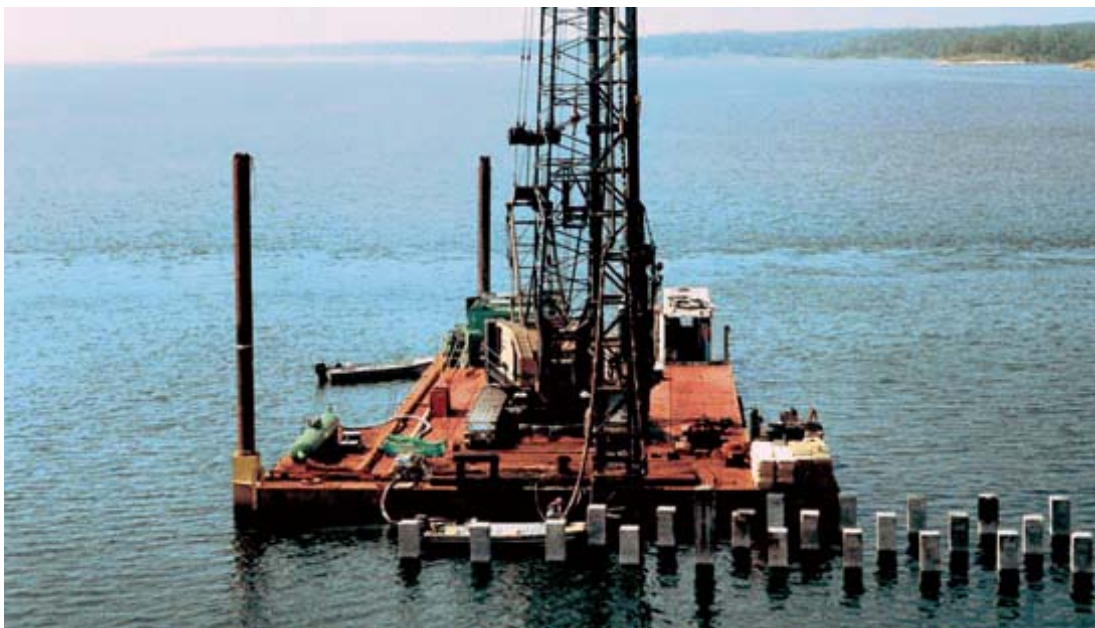
50-Ton Hookload Capacity Crane on FlexiFloat Sectional Barges
