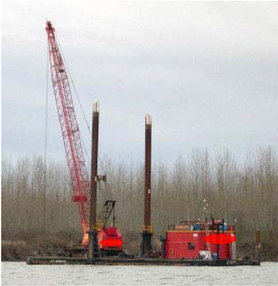
Derrck Barge - 105' x 40' x 7'-6"
