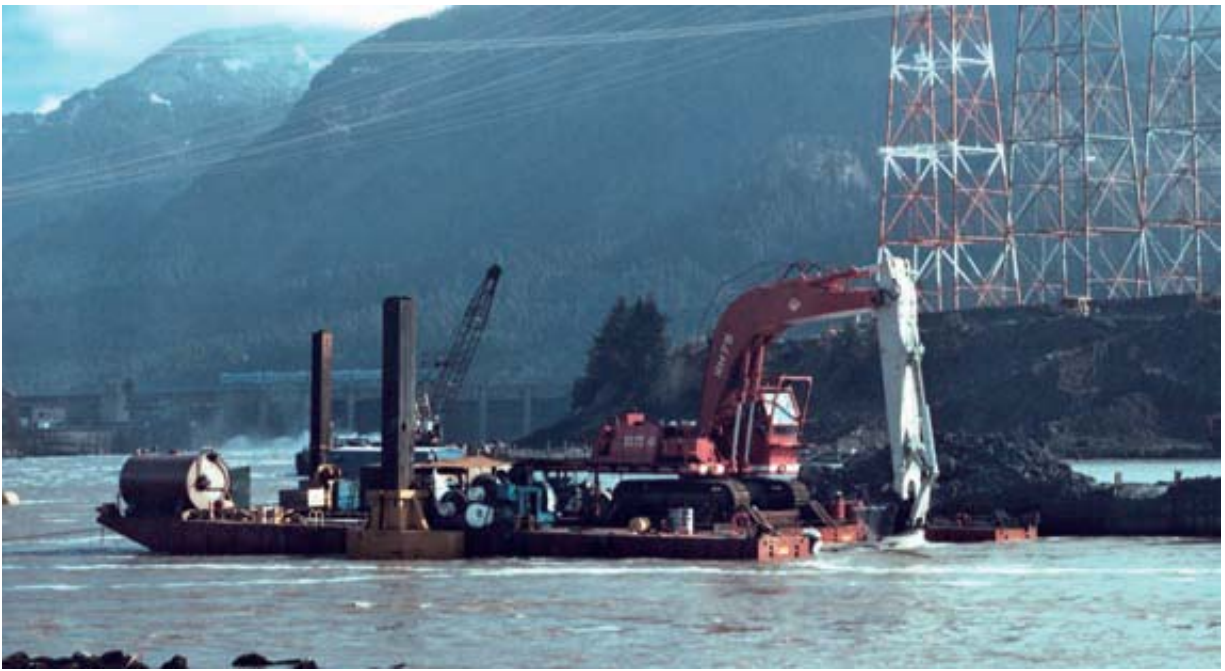
8 CY Hydraulic Excavator on Sectional Barges
