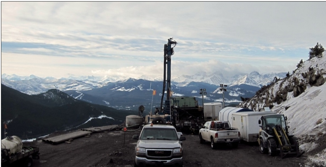
Photo B.10: Large Diameter Drill Rig on Grassy Mountain
