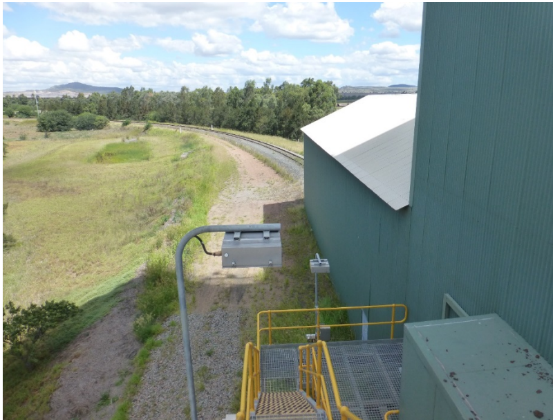
Photo 1.2-2 Bengalla Mine (Australia) Metal Clad TLO structure, illustrating the enclosed roof. The proposed TLO for the Grassy Mountain Coal Project will have a similar configuration and enclosed roof.
