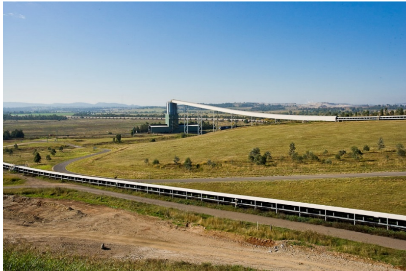
Photo 1.2-1 The existing Bengalla Mine (Australia) TLO System.
