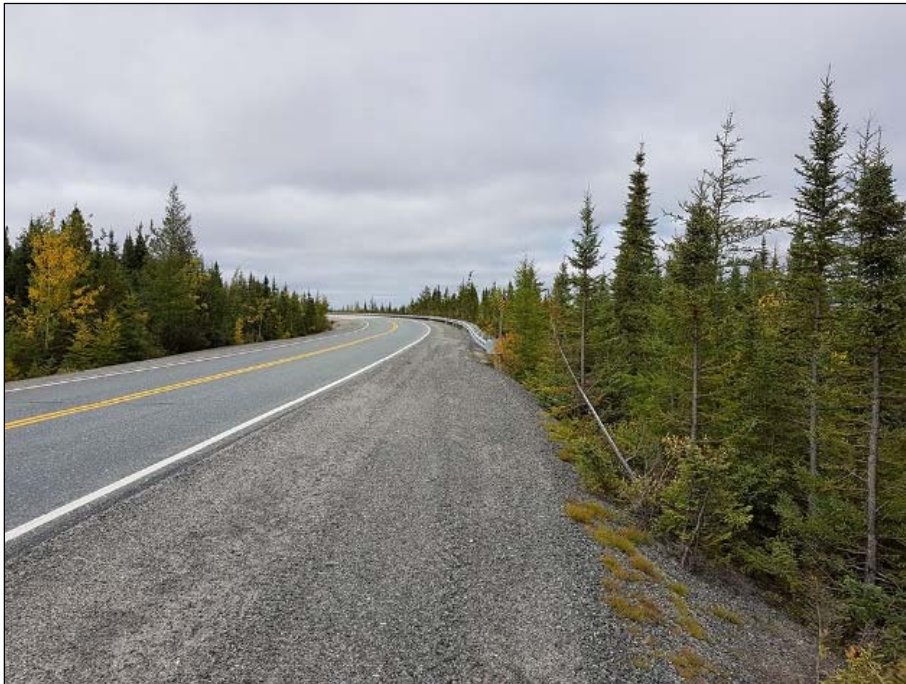
Photo 6-15 Road landscape unit
