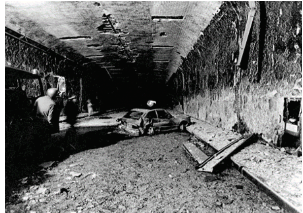
Figure 5-2: Image of the Caldecott Tunnel Fire
