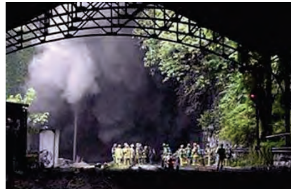
Figure 5-1: Image of the Baltimore Tunnel Fire
